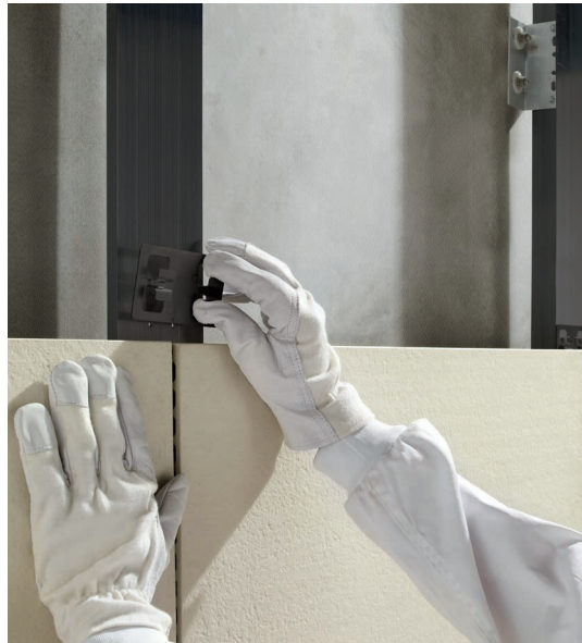
SISTEMA PLUS Anclaje con grapa FVI PLUS Attachment with clamp
