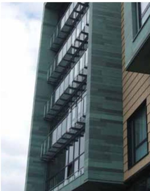
Nordic Green™ products offer designers unparalleled design freedom and the ability to determine the type and intensity of green patina for each project with choices of 'Living' surfaces. In a carefully controlled, factory process, pre-oxidised copper is treated with specifically formulated copper compounds to create the desired patina colours and heat-treated to chemically bind them to the copper.
